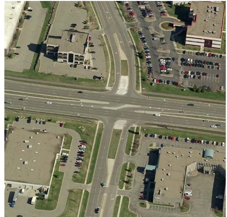
CSAH 42 at Southcross Drive in Burnsville, MN
