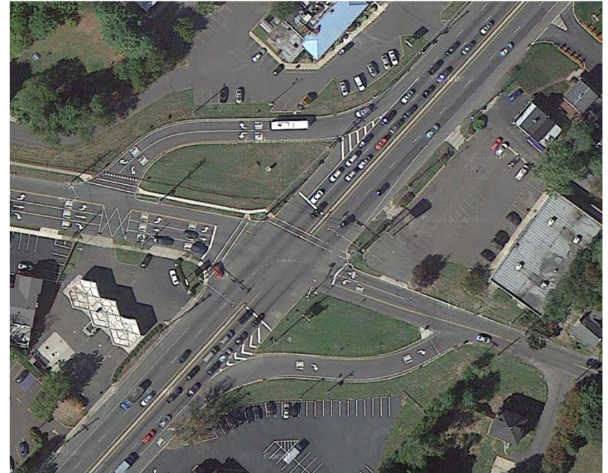
US-1 at Franklin Corner Road, Lawrenceville, NJ
